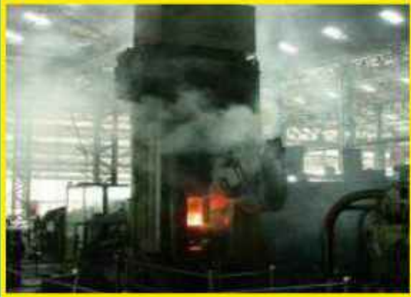
INTEGRATED SHELL FORGE PLANT
